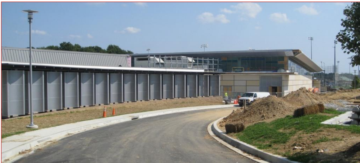
Figure 1: The facade's canopy of the Susquehanna Center is shown at the left, and the basketball arena addition is shown at the right. The photo was taken during construction in early September.
